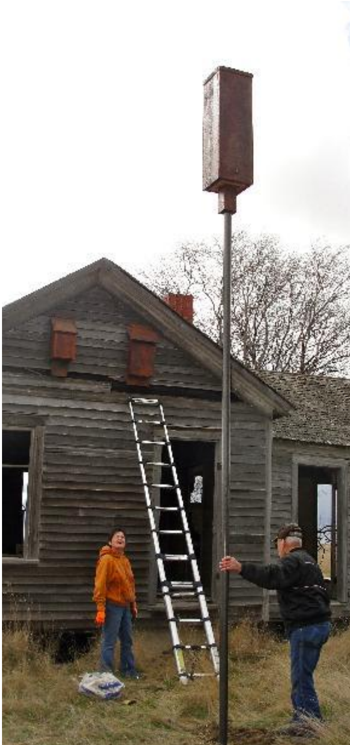
All three house designs being installed in Meadow, SD.
